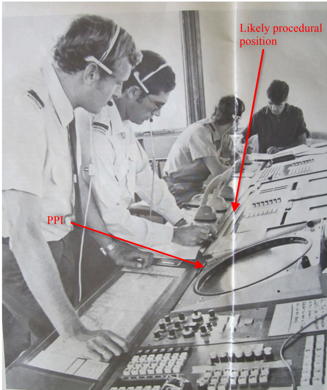
Figure 46: Williamtown control tower. As procedural control was in force, there was no permanent manning of the PPI nor was there a requirement to even have the radar on. The ATCO had to step between the procedural work area and the PPI (Photo: H. Howard c.1970's).
