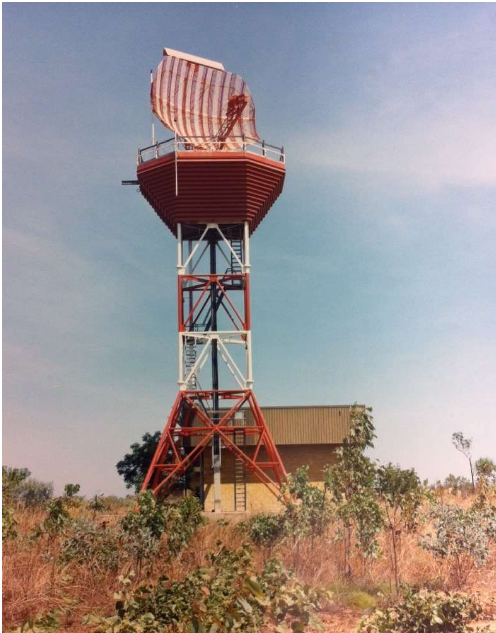
Figure 23: SURAD radar head. The PSR feed horn was estimated at being 30 meters above ground level whilst the SSR antenna was estimated at being 2 meters above the PSR feed horn. Such information is important in radio propagation studies (Photo: Australian Government (Department of Defence) c.1980).
